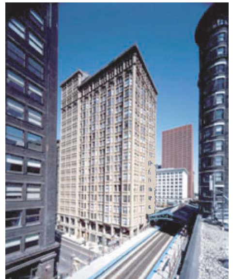
Historic Fisher Building, Chicago, Illinois Critical Facade Inspection and Facade Restoration
